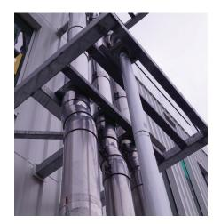
Robin was impressed with Secure Stack Pros unique self-centering design and coupling configuration that requires only one locking band and a standard, high-temperature silicon sealant for secure connection.
