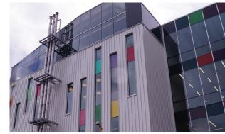
in outdoor lighting, the nearly 290,000 sq. ft. building is vibrant and modern in appearance. One would scarcely notice the five-story columns of stainless-steel exhaust stack that run up the north side of the building. If anything, the exhaust vent looks like an architectural embellishment. But make no mistake, each 61-foot column is there to serve a very important purpose.
