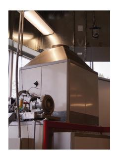
Robin instructed fabricators at Northwest Sheet Metal's shop in Surrey, British Columbia, to make stainless steel sleeves to fit around the single wall vent. Workers were able to install, as approved by Secuirty Chimney engineers, the 2-piece half-circle sleeve sections and insulation around the single wall sections after all the exhaust vent was installed. In addition, Security Chimney custom fabricated several anchor plates to accommodate the existing structural steel supports.
