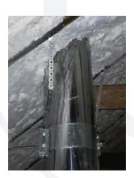
This example shows spray-foam insulation in direct contact with the chimney, which is a serious potential fire hazard!
